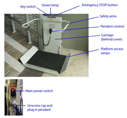
The drive unit (shown in Figure 2 below) has the following components:
